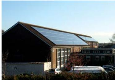
The 540-panel solar photovoltaic installation is situated over two roofs at Matthew Arnold School, off Cumnor Hill, Oxford. It consists of two arrays: a 52 kWp array on the main school block and a 48 kWp array on the science
